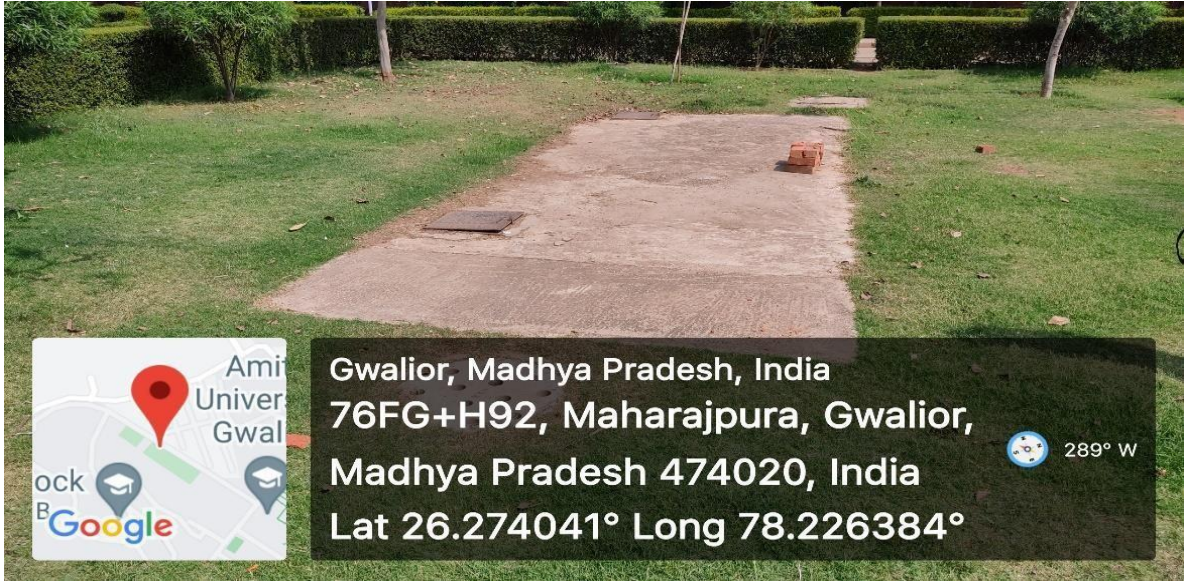
Rain Water Harvesting System A Block
