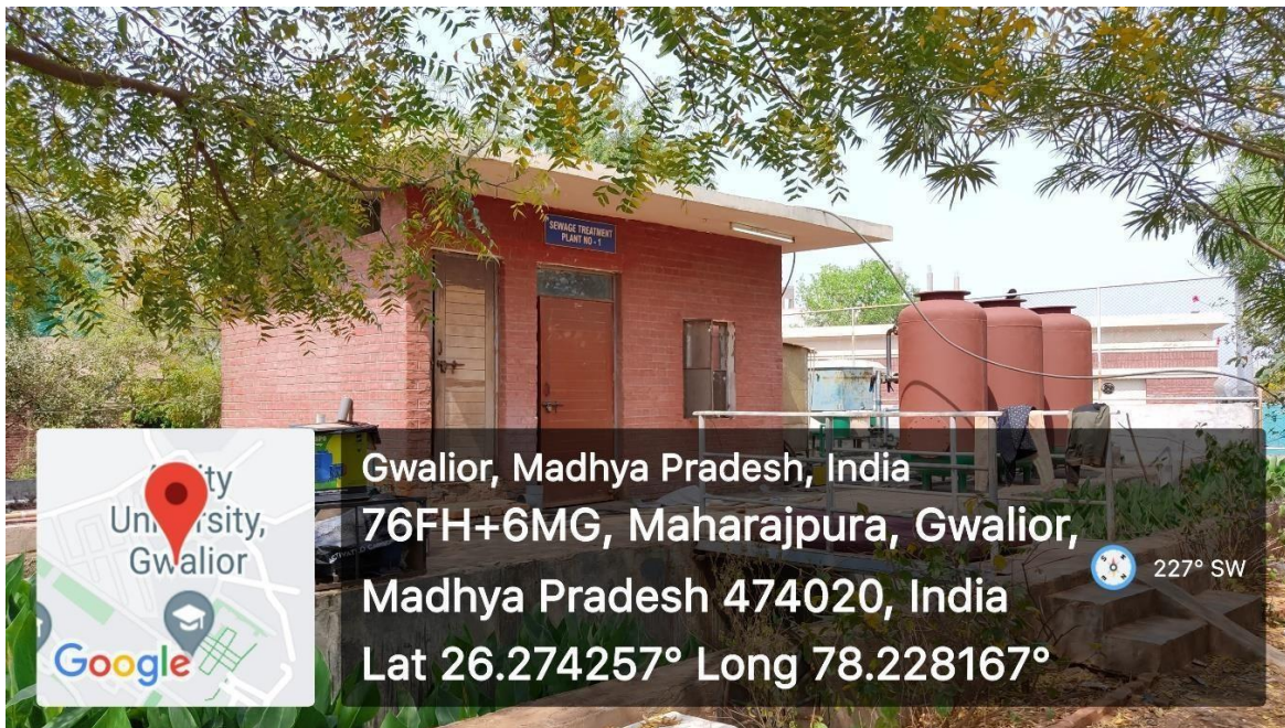
Waste Water Recycling System Near Hostel Crossing
