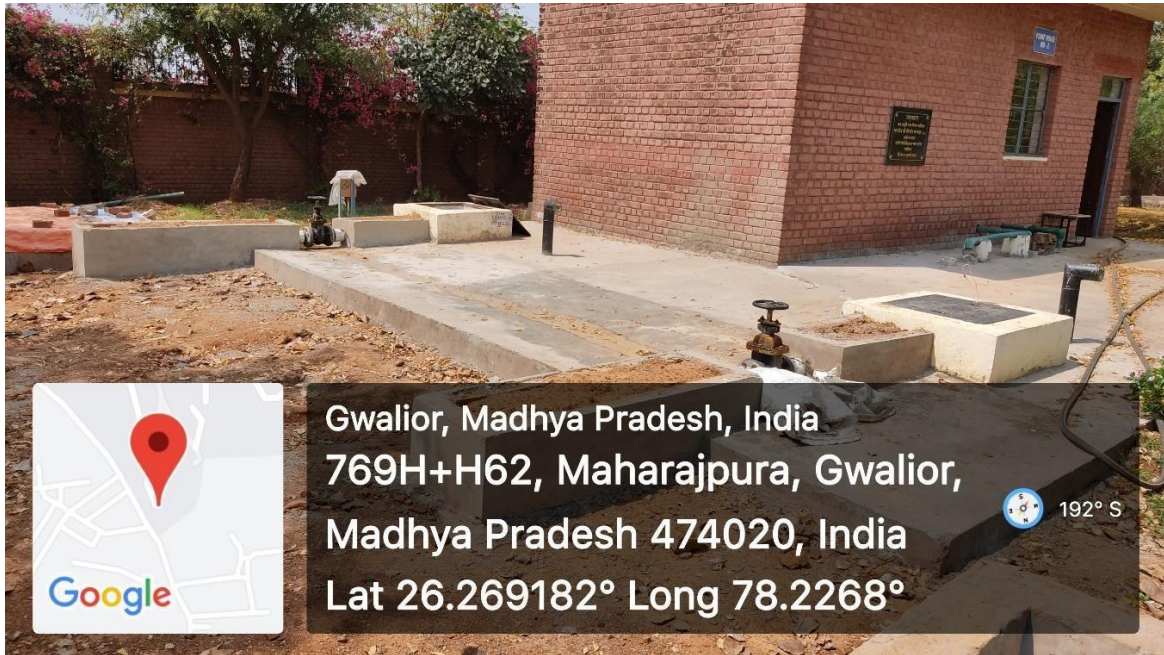
Tanks Behind C Block
